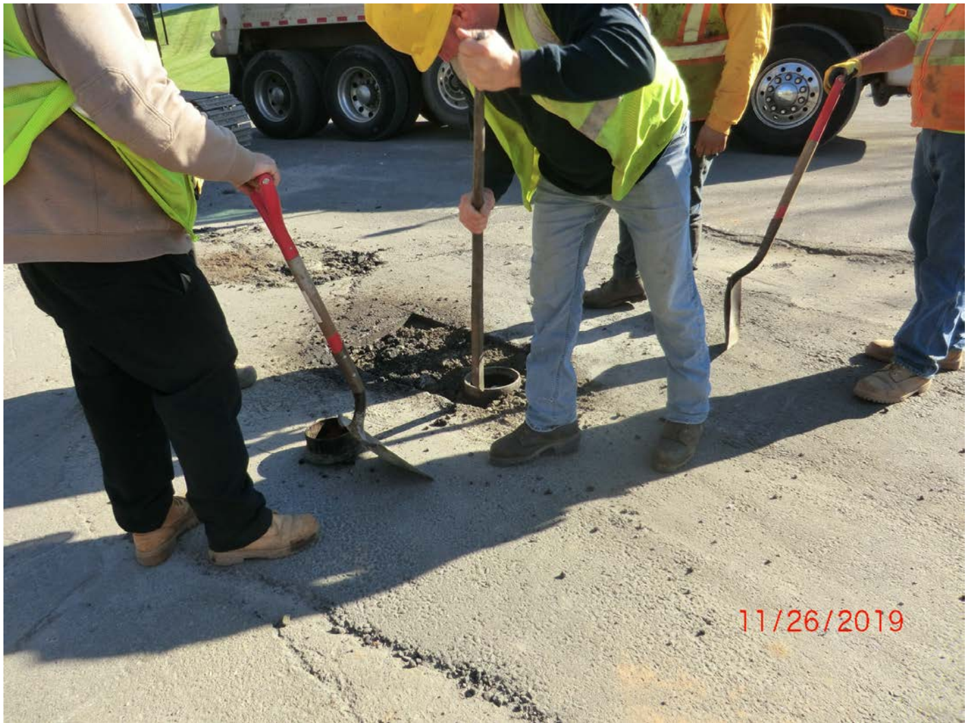
Figure 15 – ‘Shimming’ gate valve covers on Talcott Ridge. Raising structures to be consistent with road surface.
