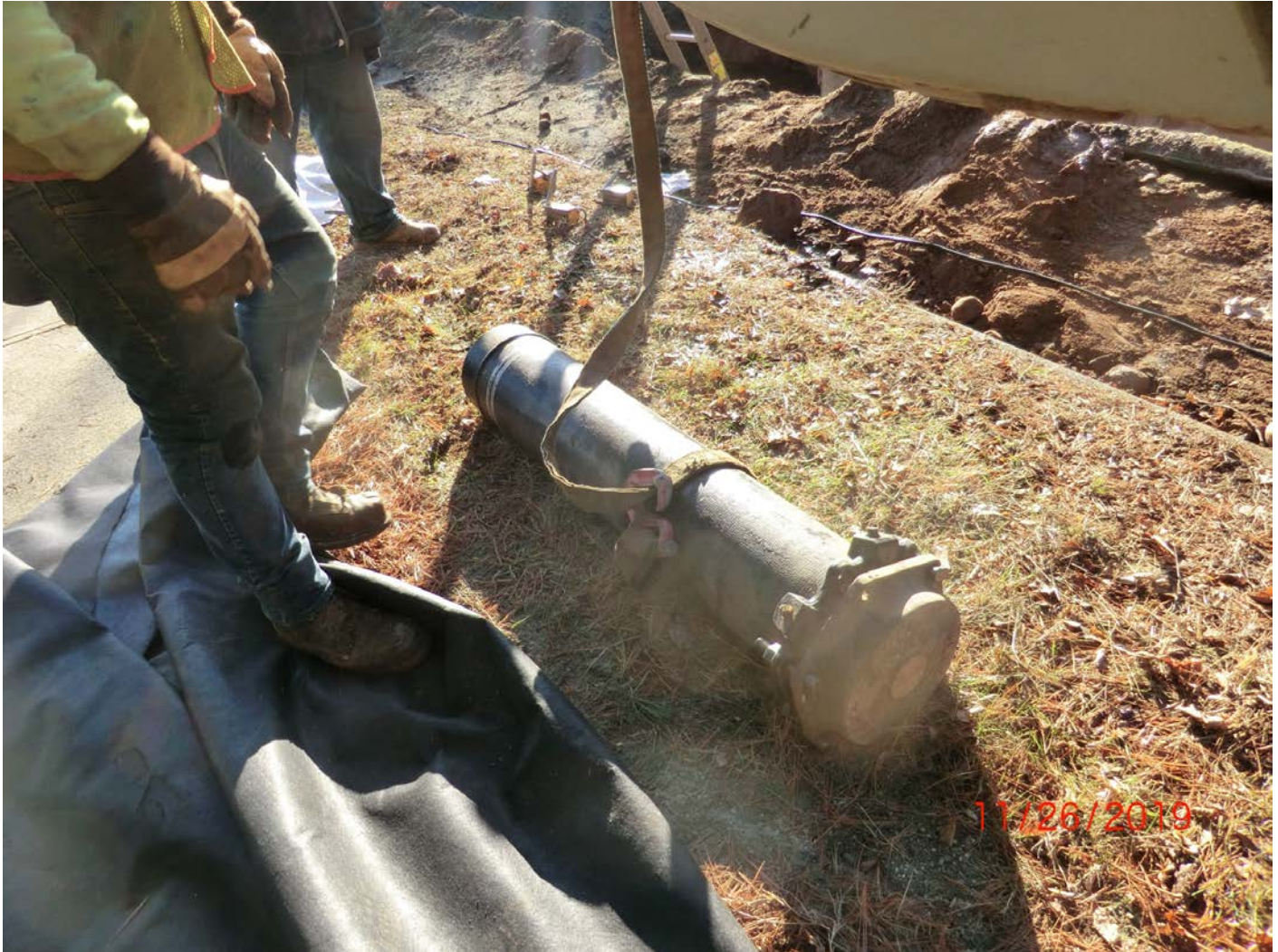
Figure 7 – 4-foot (restrained) stub installed at end of 4 th stick of 8” DI installed, bringing end of 8” DI to 752+30.
