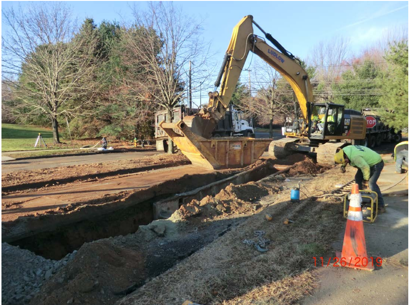
Figure 2 – Facing southwest. Morning progress towards South Main St. Note Stop Sign in background was not damaged during work activities, excavator was able to work about the sign, but ended up creating a bit of a mess to avoid damaging the sign. See later figures showing mess that was later cleaned up.
