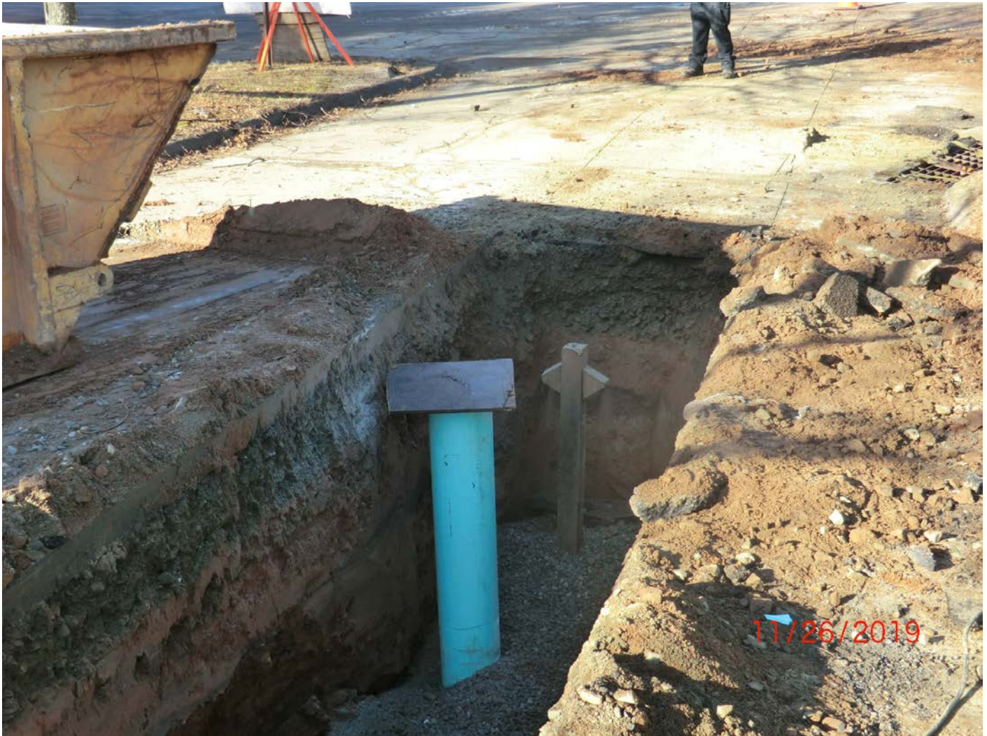
Figure 12 – End of the line 752+30. Facing west, 10'-sump and 4x4 stud at end of 4-foot stub. Starting location for next spring when 8" DIP line will extend into South Main Street. Top of picture is intersection of Talcott Ridge Drive and South Main Street in Middletown, CT.
