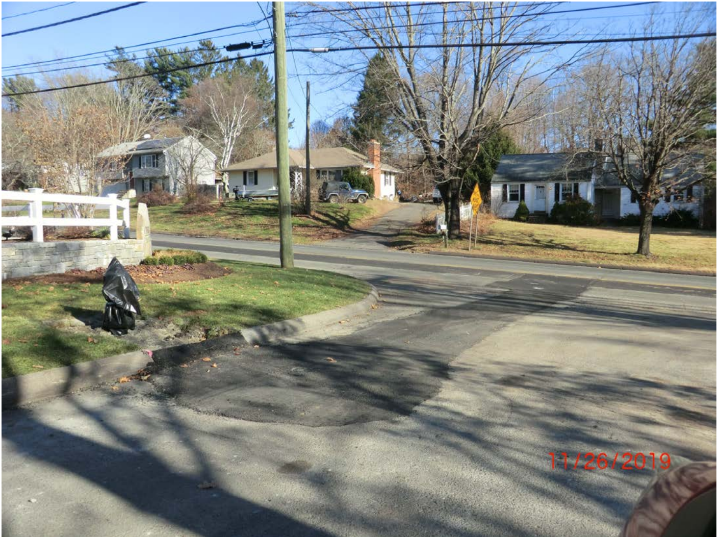
Figure 16 – New hydrant on Winsome Street, at corner with Main St., Durham, CT. Facing east-northeast.
