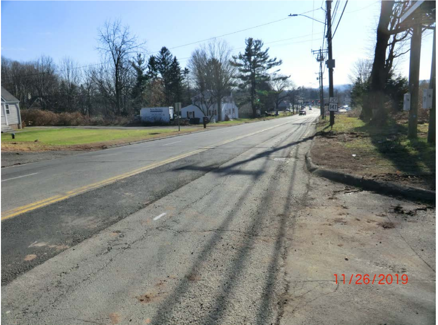
Figure 17 – Facing south, repaired/repaved trench line on Main St. Durham. Winsome St. to right of photo.
