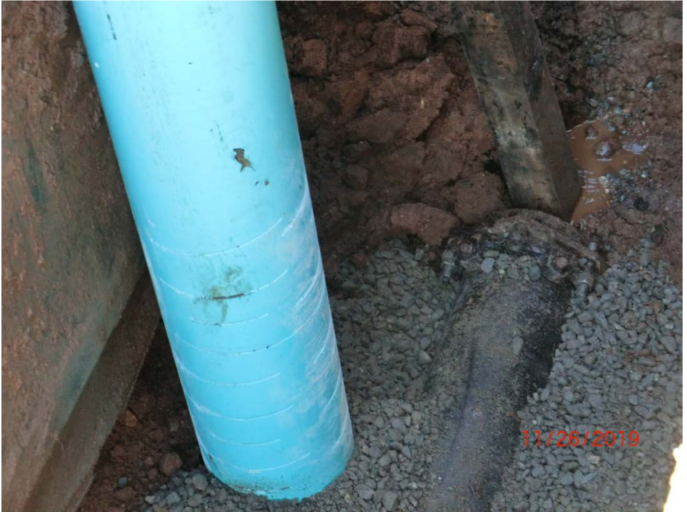
Figure 10 – Installation of 10” pipe cut sump adjacent to stub. Note 4x4 stud at top of picture marking end of todays run.
