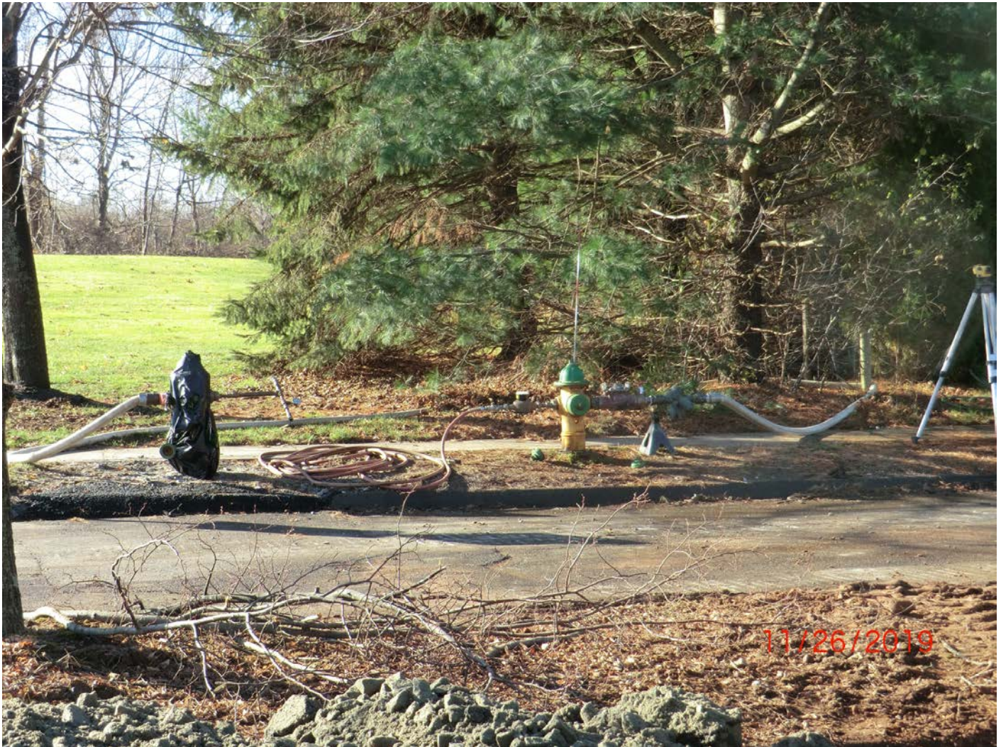
Figure 13 – Cross over from active hydrant to new hydrant. Set up was used by Peter (Ludlow) to fill the water lines going up Talcott Ridge and Watch Hill.
