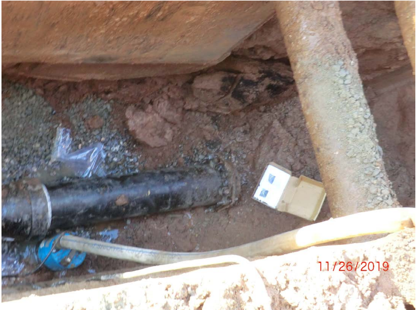
Figure 8 – Installed 4-foot stub.
