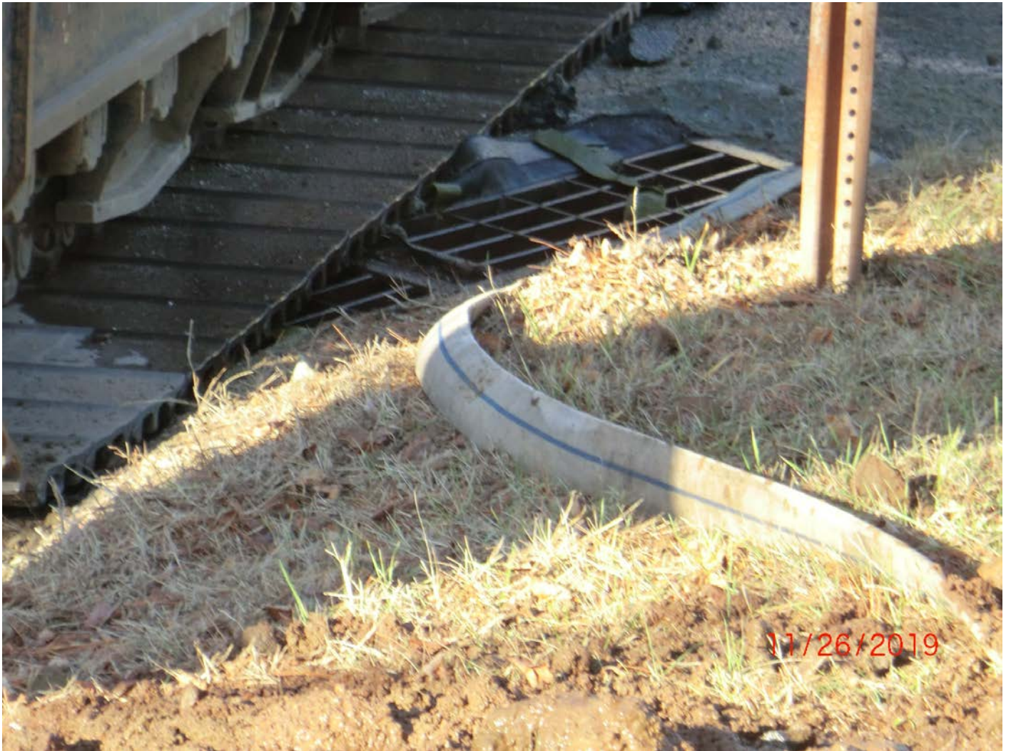
Figure 5 – Sump discharge to protected catch basin.
