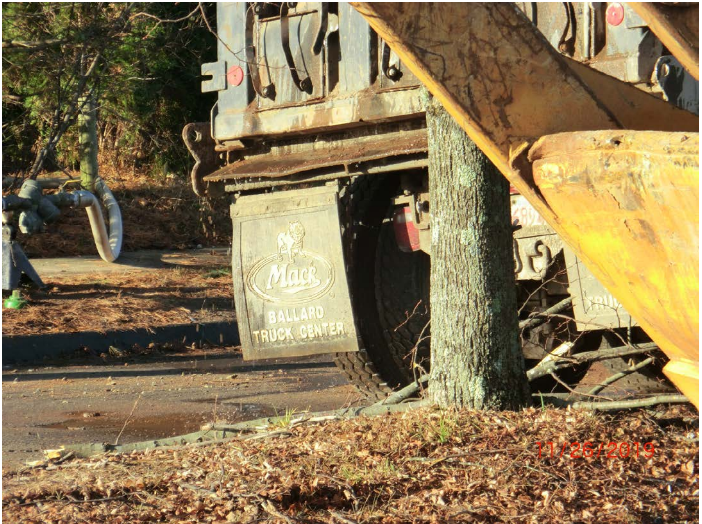
Figure 3 – Facing southwest. Having reached bottom of Talcott Ridge, the trench has again encountered the groundwater. Water can be seen here dripping from the back corner of the dump truck.
