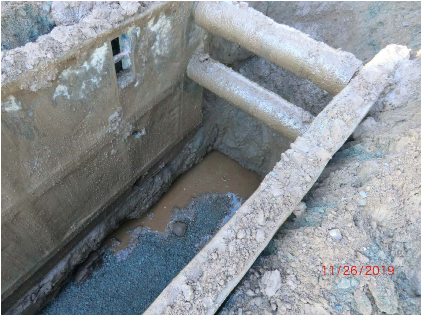
Figure 4 – Water in trench. Sump pump used to dewater to fabric (silt fenced) lined catch basin.
