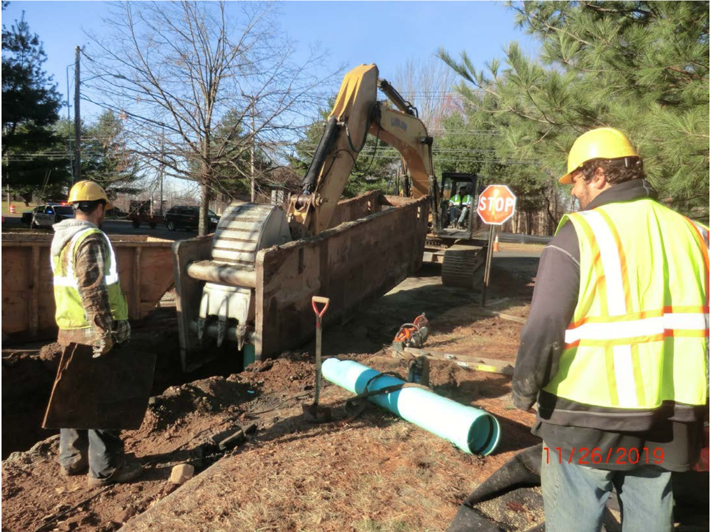
Figure 11 – Facing west. Removing 24-foot trench-box.
