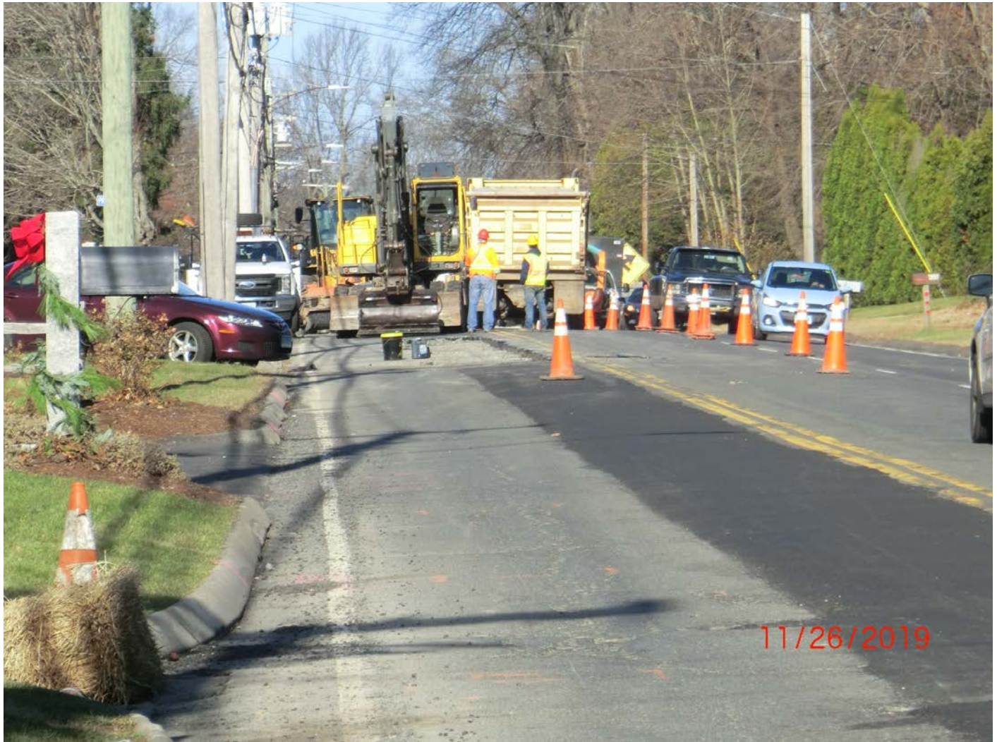
Figure 19 – Completing work at Parsons Street, installing hydrant of Tee in Main St. Water line. Picture facing north.
